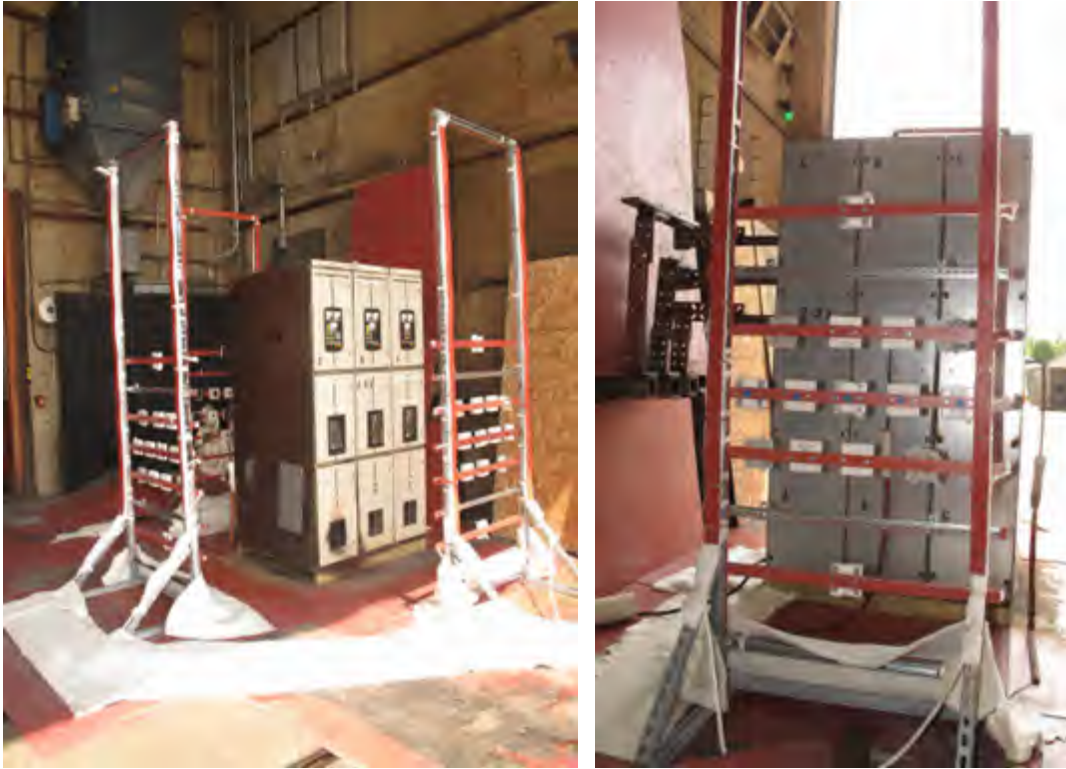
Fig. 166. Pre-Experiment 2-33B in test cell. Left – front corner view, Right – experimental device viewed from rear.
