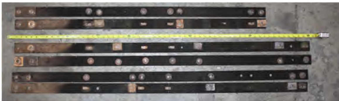
Fig. 172. Post-Experiment 2-33B Horizontal Main Bus Conductors.
