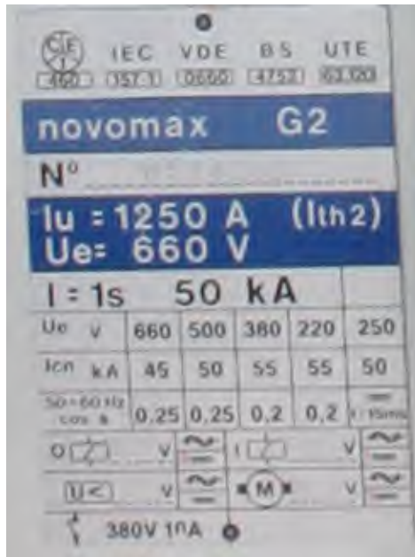
Fig. 19. Photo of LV breaker name plate
