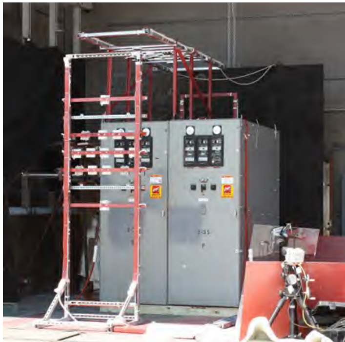
Fig. 25. Photo of instrumentation racks during experimental setup.
