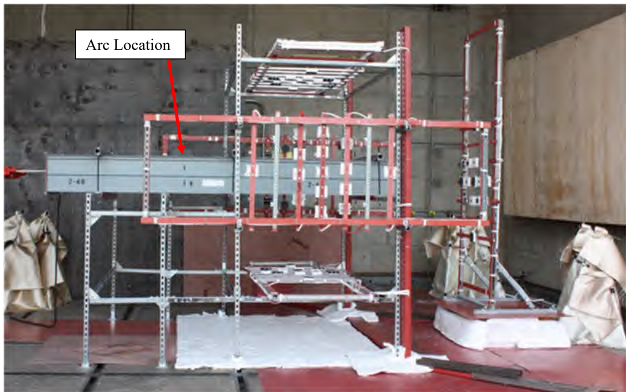
Fig. 201. Pre-Experiment 2-40 Bus Duct. Duct and instrument rack configuration prior to experiment, arc initiated at arrow.
