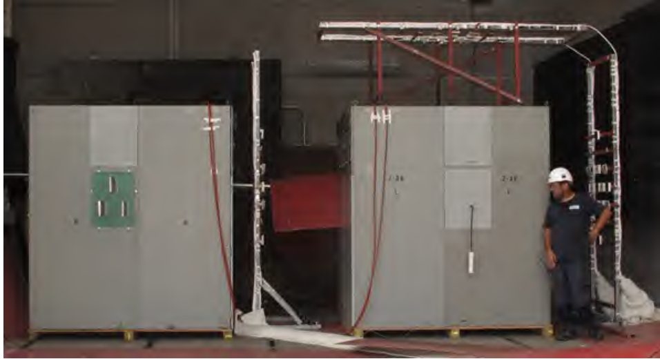
Fig. 191. Pre-experiment 2-38 Enclosure “M” and “L”. Front view of “cross-aisle” configuration. Arc initiated in Enclosure “K” located behind Enclosure “L”.
