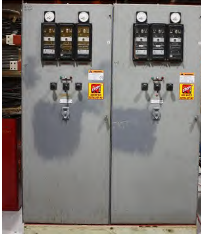
Fig. 12. Type M-36 Metal Clad Enclosure. Enclosure “O” shown left, “P” shown right. (note: bus bar extensions shown left, and breaker not shown)
